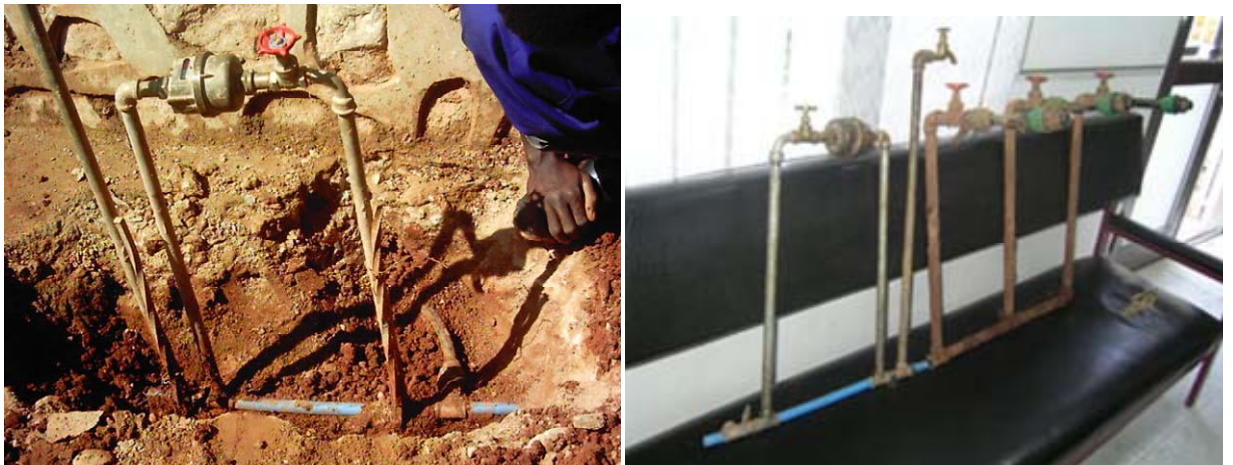
Plate 1: Examples of meter by passes in the field
