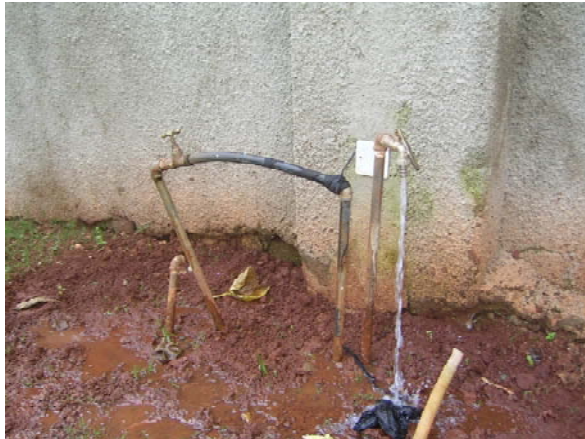
Plate 3a: A connection that allows a customer to fetch water before the meter and b) An example of what a reversed meter shows
